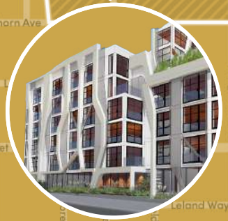
Hollywood Cherokee nears completion
